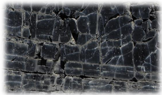
A DAMAGED SECTION OF OBSIDIAN WALL
